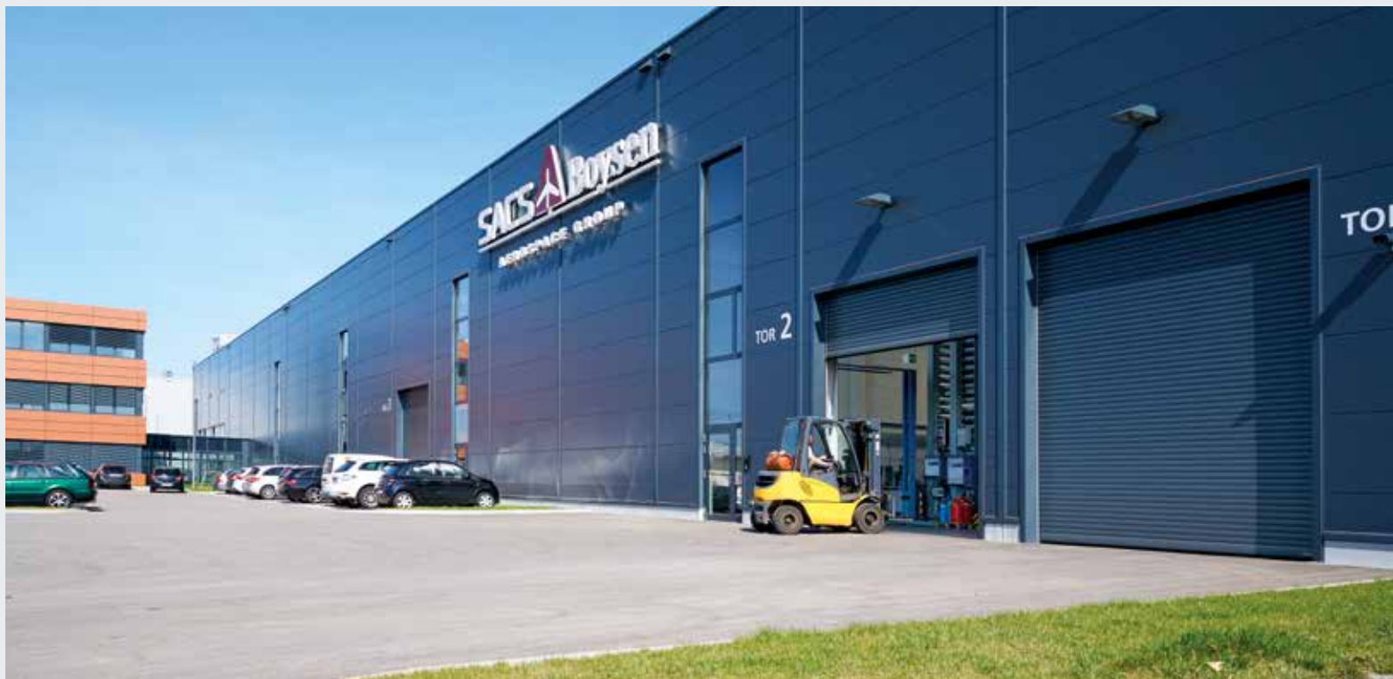
The standard light grille at the side guides reduces the risk of collisions with forklifts.
